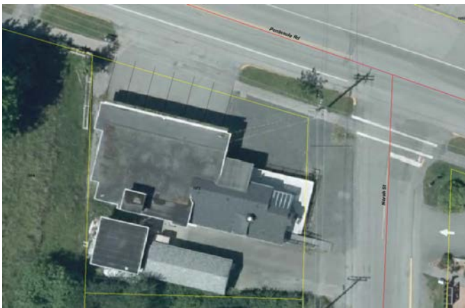
Figure 3 – Existing parking for Subject Property
